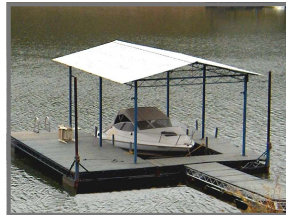
Single slip party dock on a deep water cove will never run out of water!
